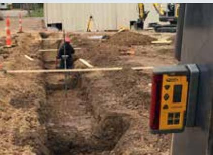
The Spectra Precision® CR700 Combination Laser Receiver is a machine mounted display receiver used on small grading and excavating equipment as well as a traditional laser receiver mounted to a grade rods. It is also ideally suited to work in vertical applications for alignment control.
